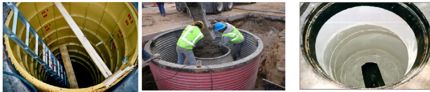
Figure 5 . Example Applications of Manhole Rehabilitation using FIP Methods
