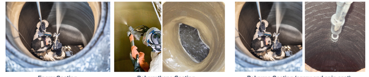
Figure 6 . Manhole Rehabilitation Using Polymer Coatings (Epoxies, Polyurethanes, Polyureas)
