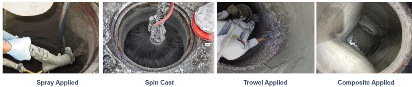
Figure 4 . Example Rehabilitation Methods Using Cementitious Technologies
